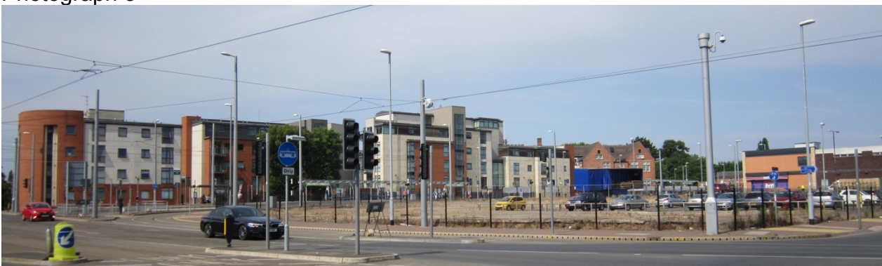
Styring Street site Station Road
